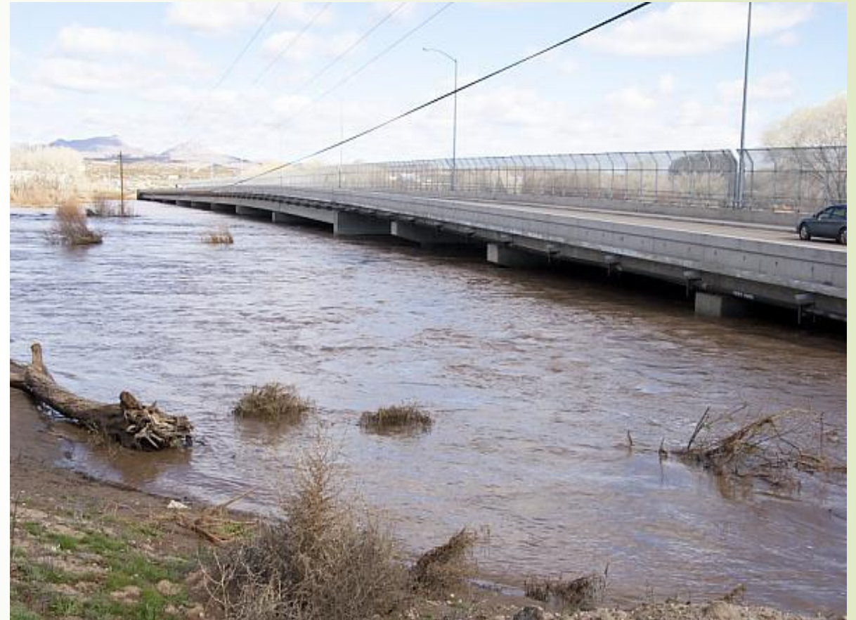
Figure 3: Bridge Crossing the Gila River in Duncan, AZ [2]
